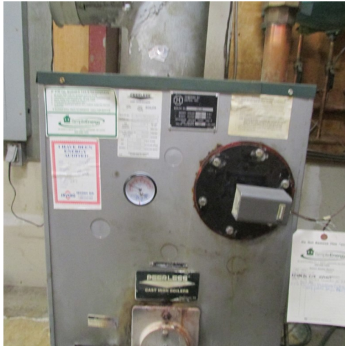
Peerless Oil Boiler Model EC(T)-06-275m/S Manufactured December 1999 DOE Output 321KBtu/Hr Net IBR 279KBtu/Hr
